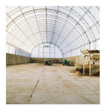
Being a highly corrosive material, fertilizer requires a durable storage solution, protected against deterioration and harsh weather conditions. With sustainable materials and reduced installation time, this was the optimal fertilizer storage solution.
